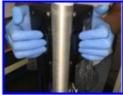
Attach Control Module To Utility Pole
